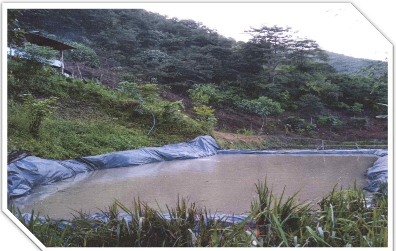
MAKASEM WATER BODY USING POND LINERS AT TUENSANG VILLAGE
