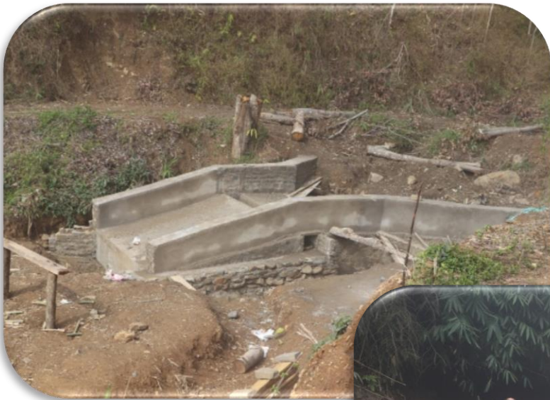
Trench Weir 1 and Trench Weir 2 under construction
